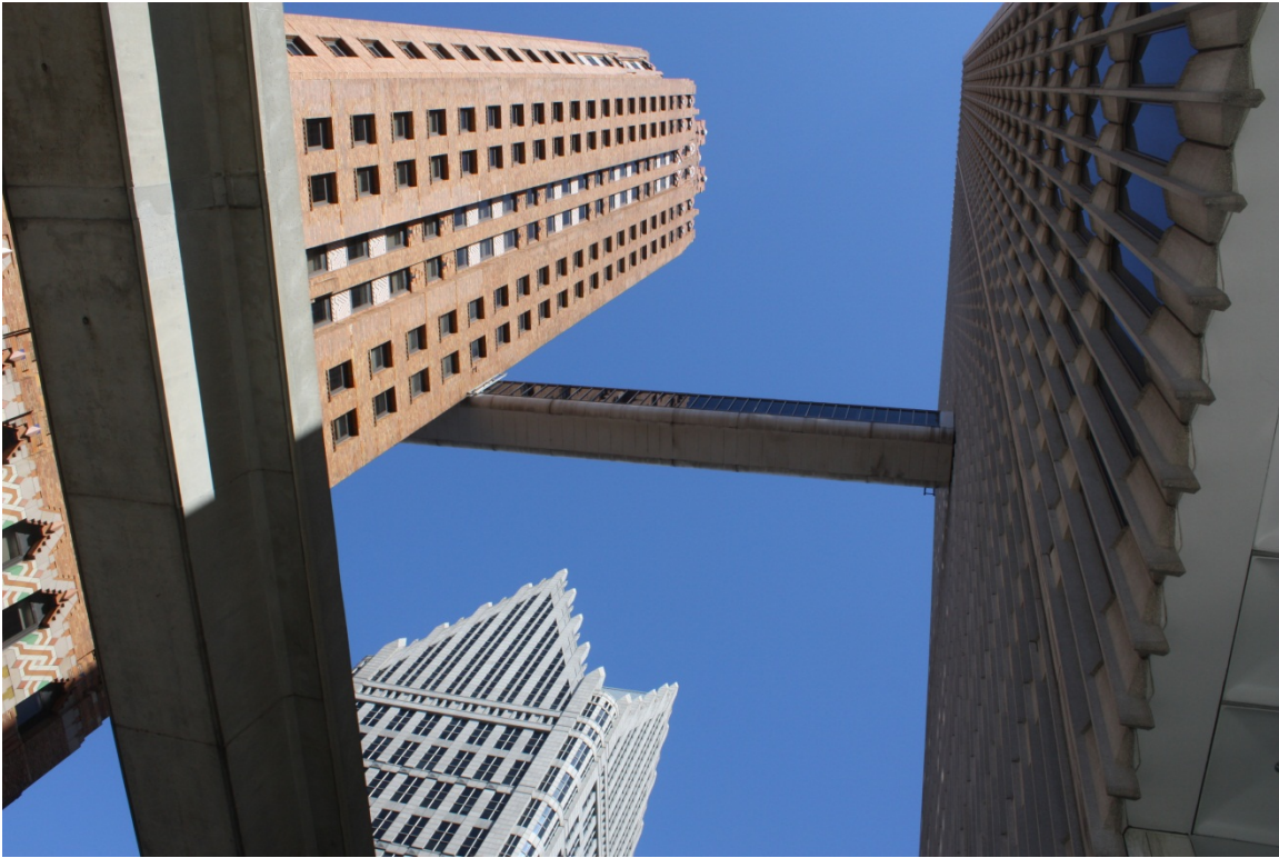
The Detroit People Mover connects downtown's architectural gems.
